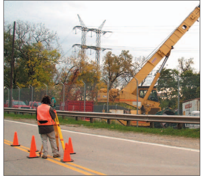
KS Associates provides surveying services to support shaft site construction.
